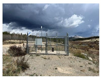
single-phase motor. The pump intake depth is 105-feet and the screened interval depth is 98-feet to 197-feet. Well #1 has a reported sustainable pumping rate of 70 gpm, based on pump tests conducted in 2020, however, Well #1 has recently shown a steady decline in production, when operated for sustained periods of time. The well has never been redeveloped or rehabilitated. No issues have been reported with the pumping equipment.
