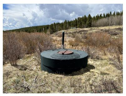
The infiltration gallery is located approximately 900-feet north of the WTP. The infiltration gallery was constructed with the WTP in 1991 and includes a 24'-2"-deep manhole, 197-feet of slotted 12-inch dia. PVC pipe, and an 18-inch dia. butterfly valve located in the manhole to control flow to the WTP. The infiltration gallery is connected to the WTP by an approximately 900-foot long, 18-inch dia. ductile-iron
