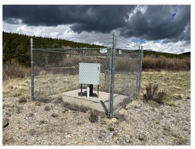
Well #2R is located south of Well #4 near the northeast corner of the pond on the WTP property. The well appears to be the second redrill of the original Well #2. Well #2R was constructed in 2007 and has a completed depth of 50-feet. The well is permitted for 300 gpm and includes a submersible pump operated with a 5 horsepower, single-phase motor. The pump intake depth is approximately 49-feet and the screened interval depth
