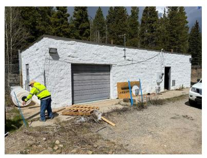
The WTP is located off Beaver Creek Road approximately 1.4 miles north and west of the Town limits. Wells 1, 2R and 3R, located on site, pump to the plant for treatment prior to distribution. Treatment at the facility includes sodium hypochlorite treatment. The well pumps supply the pressure to convey the water through the WTP to the 0.5-MG storage tank.
