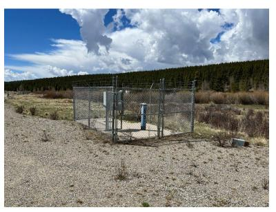
Well #3R is located north of Well #4 at the north end of the gravel access road east of the pond on the WTP property. The well is a redrill of the original Well #3. Well #3R was constructed in 2007 and has a completed depth of 65-feet. The well is permitted for 150 gpm and includes a submersible pump operated with a 5 horsepower, single-phase motor. The pump intake depth is approximately 53-feet and the screened interval depth
