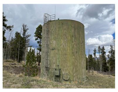
The Heights storage tank is located at 943 Quarry Road in the Beaver Ridge subdivision. The Heights tank. The welded steel tank was constructed in 1991 and has a capacity of 150,000 gallons. The tank is 28-feet in diameter and 32-feet tall. Water is supplied to the tank by the Second Street pumping station. The tank only supplies water to the Fairplay heights neighborhood. The tank was last inspected by divers in 2022.
