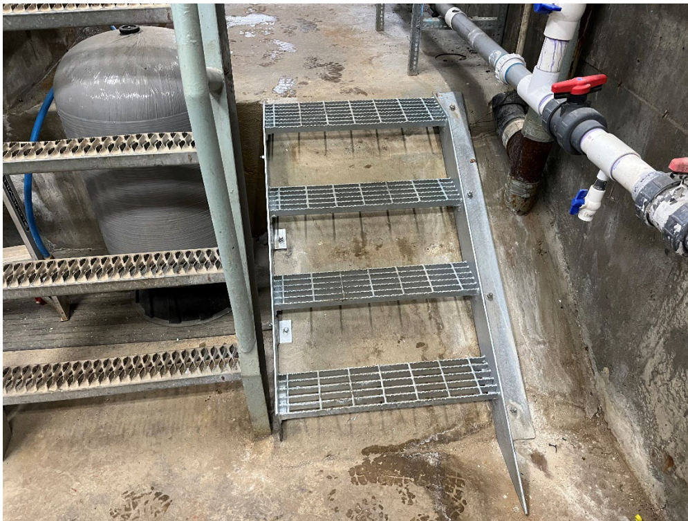
New metal grating stairs
