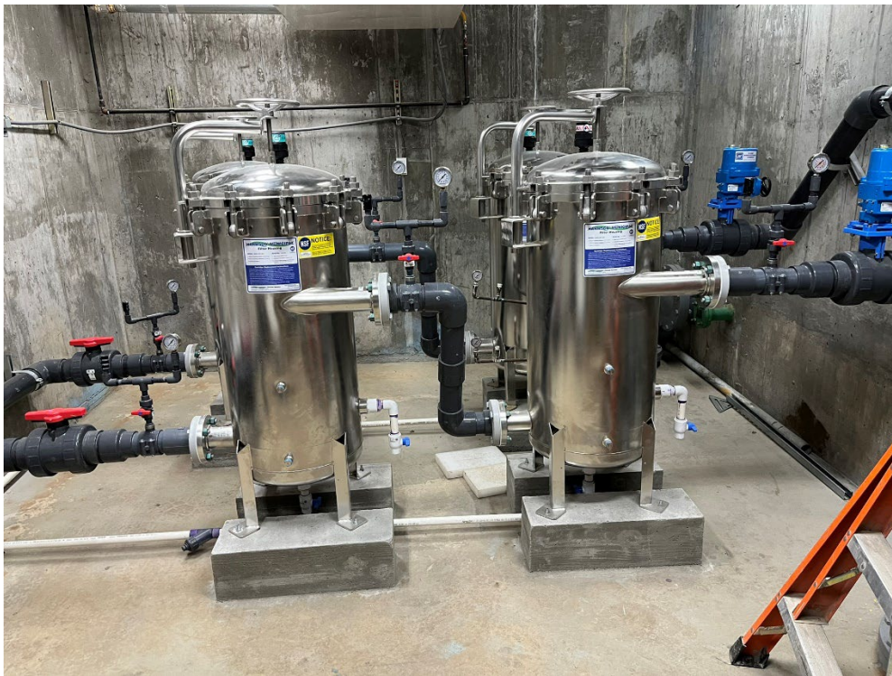
New cartridge filters installed.
