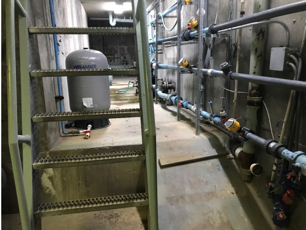
Old concrete ramp with 2x4 steps nailed into the concrete
